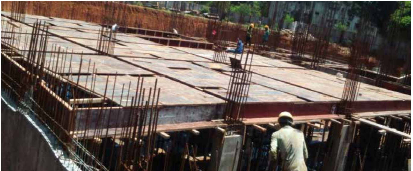
Ground Floor slab framework in progress
