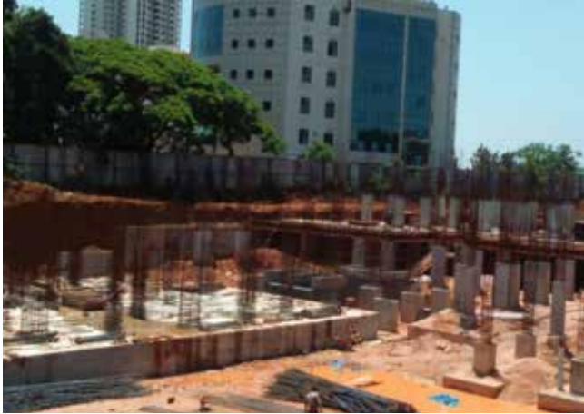
Full view of site
